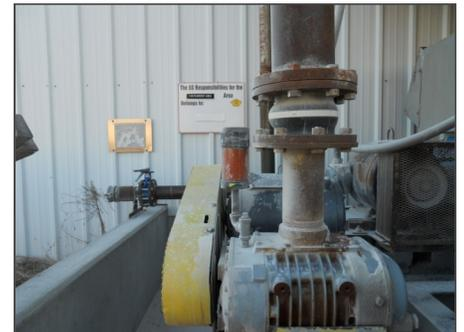
After the plant survey, Air Sentry® X-100 breathers were installed on all gearboxes. A series of third party water and particle tests confirmed the reduction of contamination below ISO cleanliness standards. Scheduled replacement of lubricants was cut back from twice a year to only once a year. This resulted in a savings of lubricant costs by more than 50% in the first year.
